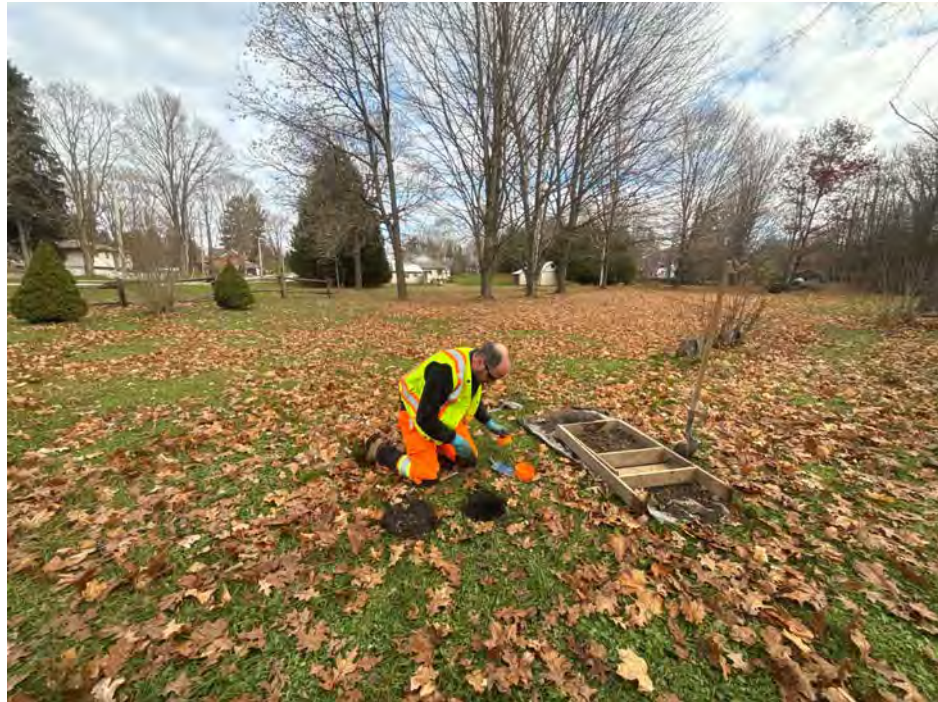
Plate 20: Fieldwork in progress; looking north
