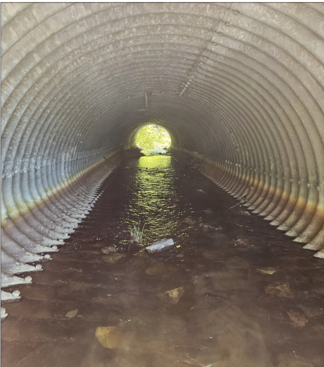
Photo 3 - View of Barrel Facing East.
