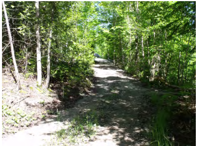
Plate 6: Looking up the driveway showing cut either side, and general slope in this area; facing NW (Photo 7496).
