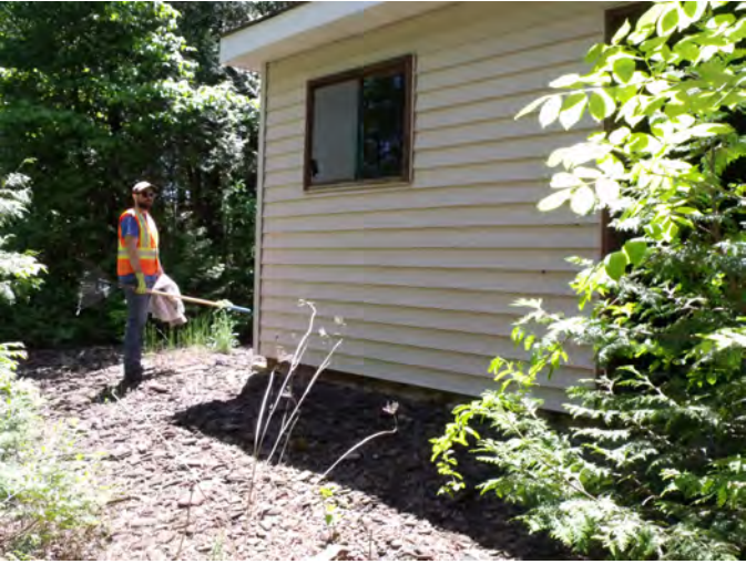
Plate 15: Structure at southern end of Study Area, showing conditions; facing SW (Photo 7539).
