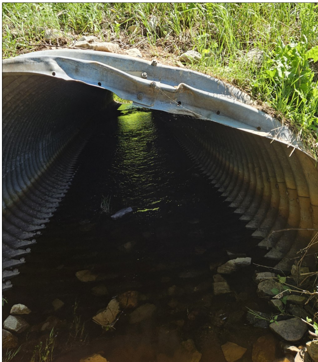
Photo 3 - View of Barrel Deformation.
