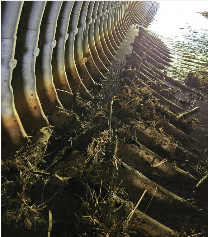
Photo 5 - View of Separation Within Culvert.
